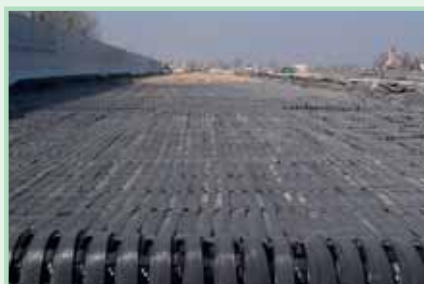
Soil reinforcement and consolidation with strip bonded geogrids in polyester fibers coated in polietilene (Paragrid® and Paralink®).
