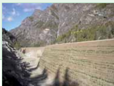
Reinforced soil structures with Terramesh® System made from double twisted wire mesh units with a stone or vegetated face.
