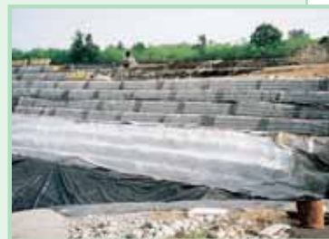
Soil reinforcement and consolidation using woven geogrids made with high tenacity polyester encased (MACGRID WG®).
