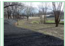
Slope and bank protection with geomats with geomats (Macmat® type) eventually reinforced during production with double twisted wire mesh or geogrids.
