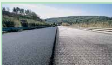
Flexible pavement reinforcement made from double twisted wire mesh incorporating transverse steel reinforcing rods (Road-Mesh® type).
