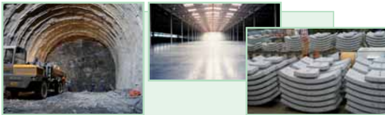
Rigid concrete pavement and tunnel reinforcement with steel wire fibres.
