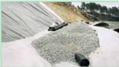
Filtration, separation, drainage and consolidation of earthworks using non-woven and woven Terram® geotextiles.
