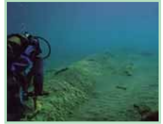
Submarine pipeline stabilisation and protection with a bituminous mattress Sarmac externally coated with a geotextile.
