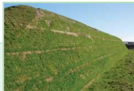
Reinforced structures for safety and /or noise barriers with Duna System®
