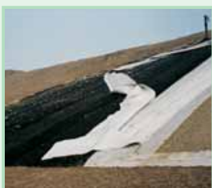
Macline® Geosynthetic clay liner (with natural sodium bentonite) for waterproofing of landfills, channel linings and basins.
