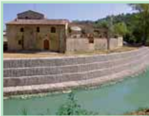
Retaining walls and river training works with double twisted wire mesh gabions filled with stones eventually combined with plants for the realizations of bioengineering Techniques.
